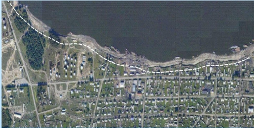
Shoreline of the Ob river at Kargasok (white dotted line shows the forecasted change of the shoreline by 2010) (Source: Krutovskiy, 2000)
